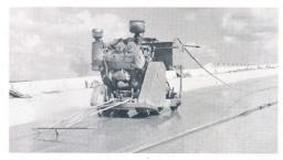
60.5-hp V-461D on concrete saw
